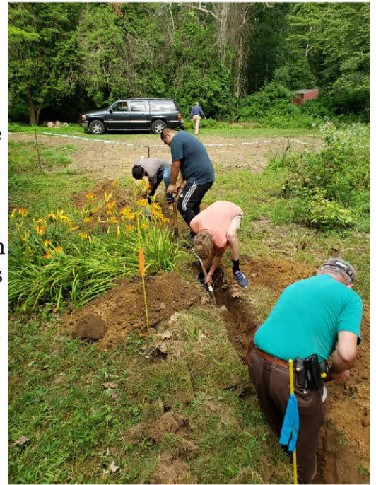
Students and Phil digging ditch for irrigation piping at Deborah's Garden
